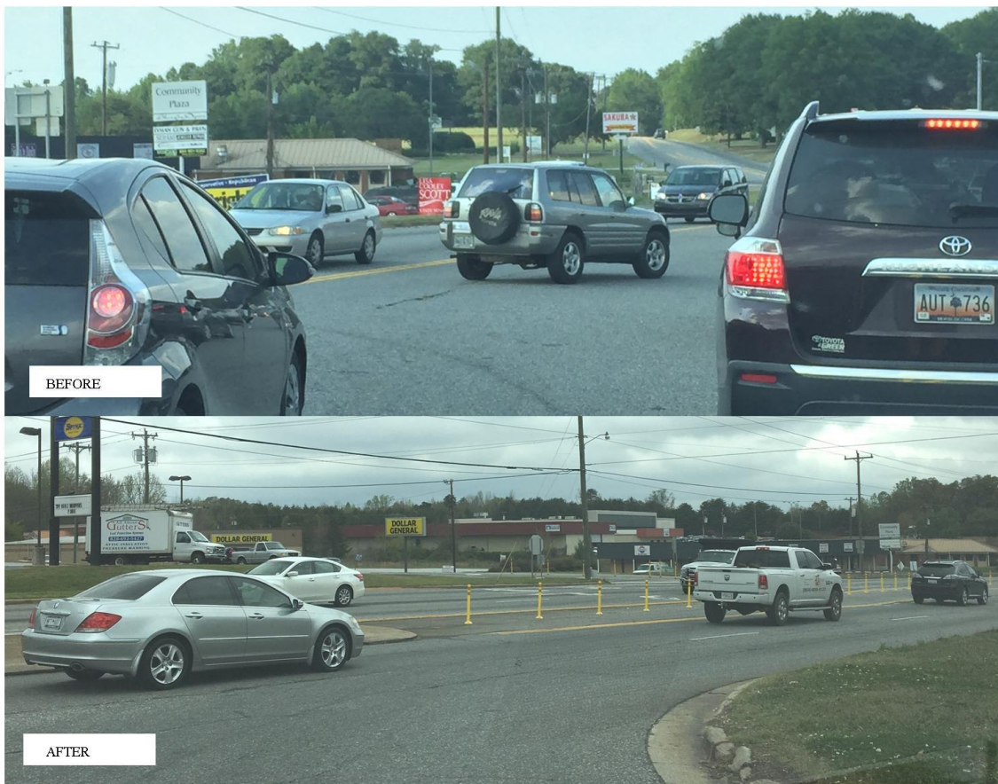
Example of Access Management and Safety Improvements- Intersection of US 29 and SC 129 in Lyman
